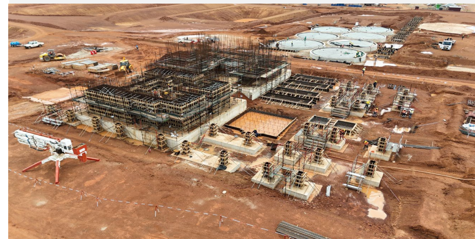
Process Plant- Milling Area – Civil/Concrete Construction
