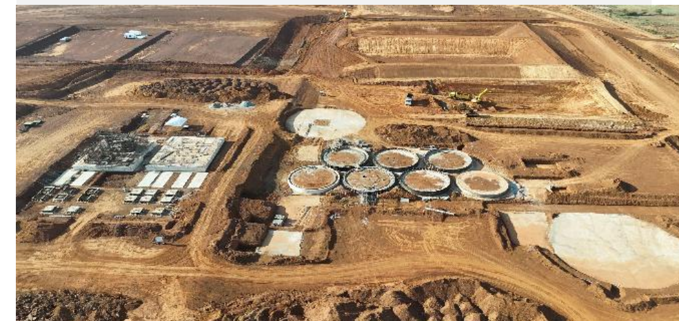
Process Plant civils works
