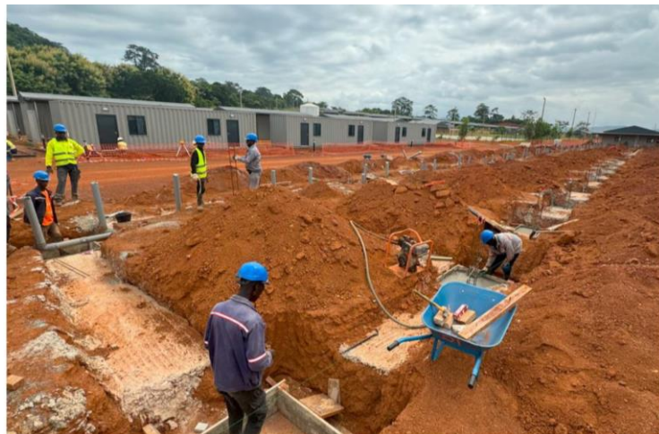
Early Infrastructure Camp Buildings Foundations
