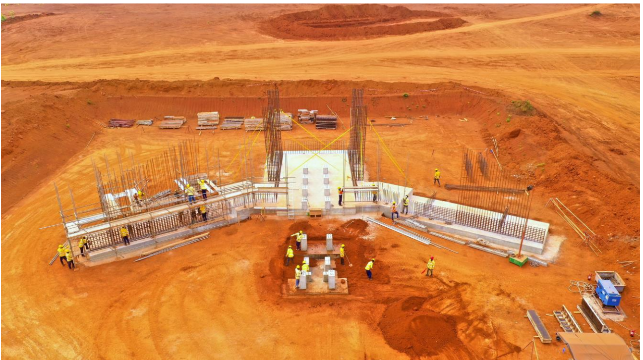
Primary Crusher Foundations
