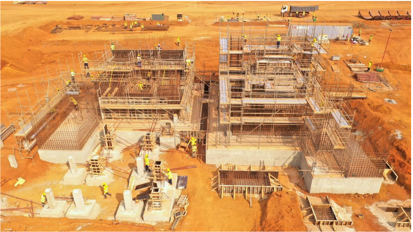
Ball and Sag mill foundations and support structure
