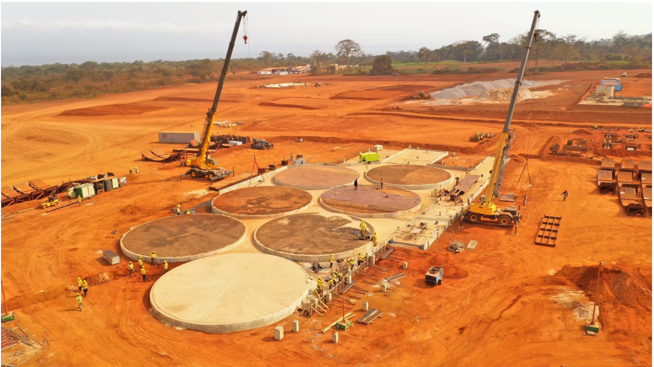
CIL Tank foundations
