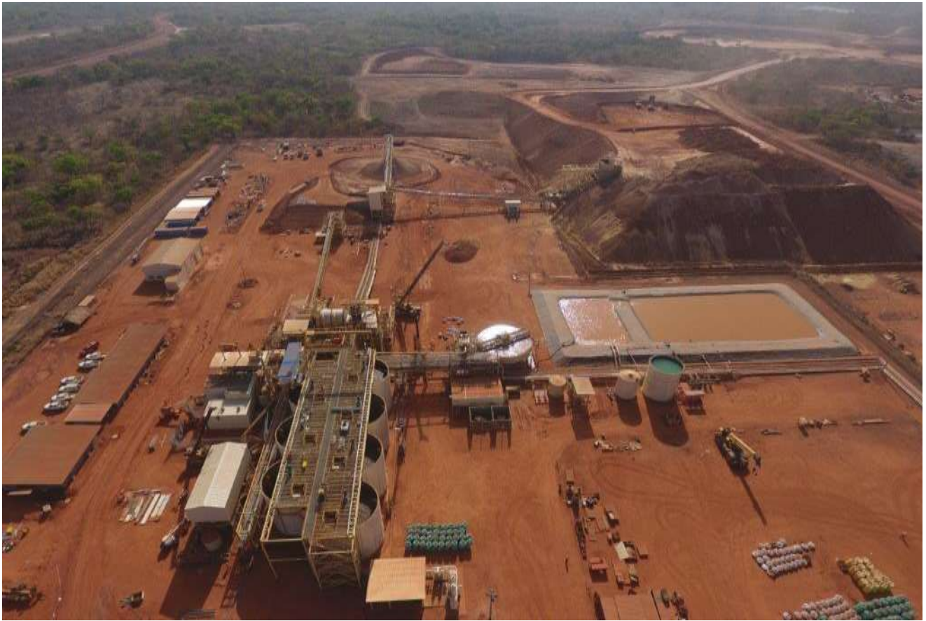
Aerial view of Sissingué Plant site
