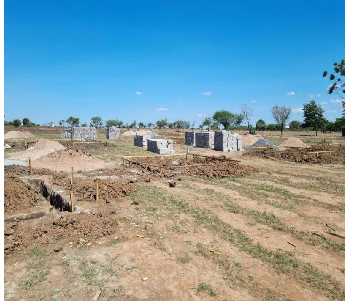
Bridgeman Nyabilla Project Area C _Footing / Excavation
