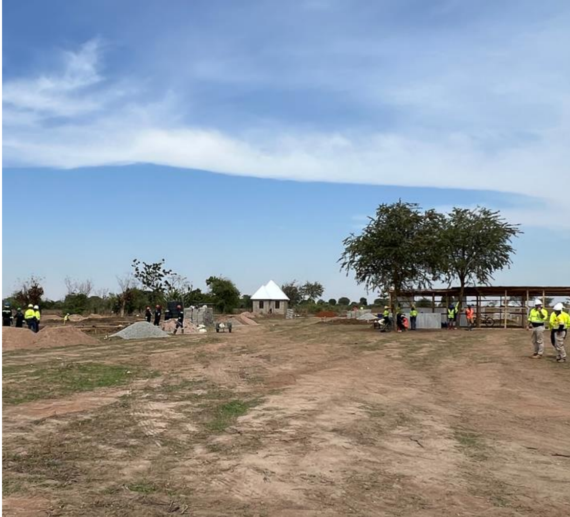
Bridgeman Nyabilla Project Area C – Site Inspection / Area Control
