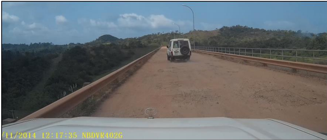
Figure 3.6: Road to the Dam
