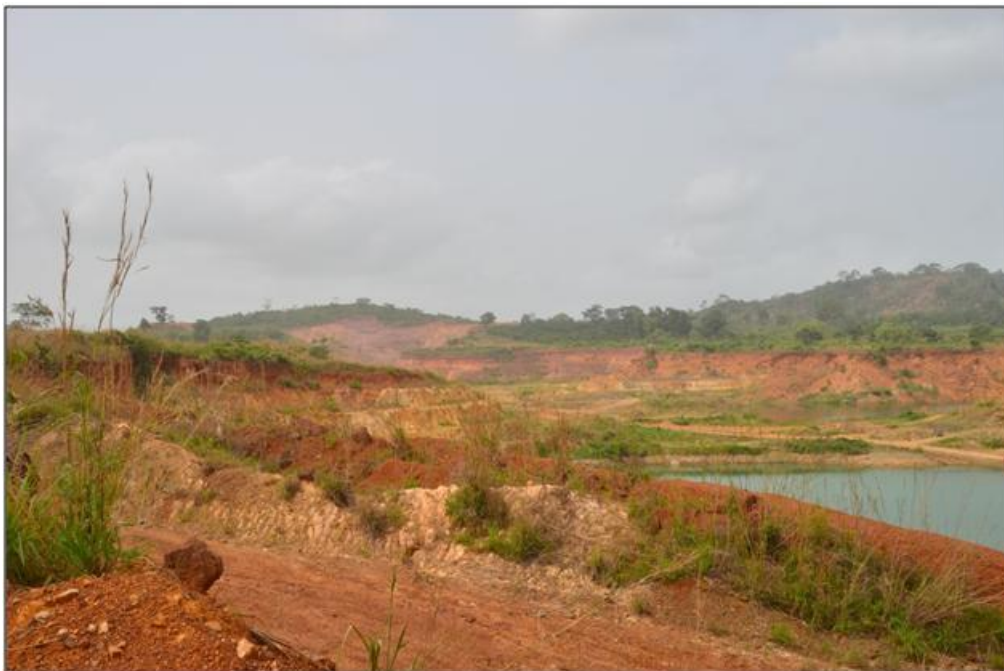
Figure 3-10: Existing mining activities within the northern section
