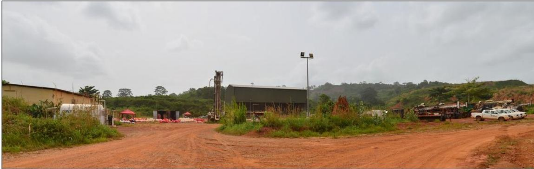
Figure C-2: Current mining infrastructure: View towards the east
