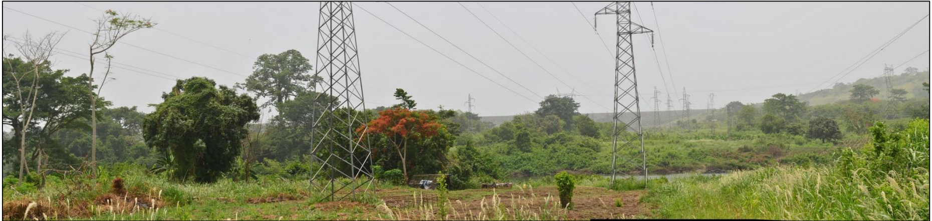
Figure C-12: Power lines from Kossou hydroelectric power station: view in a north-eastern direction
