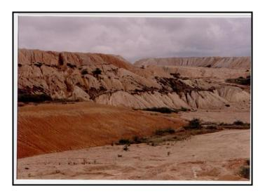
Photo 1.38 Unreclaimed Heap Leach Pad (Phase not specified)
