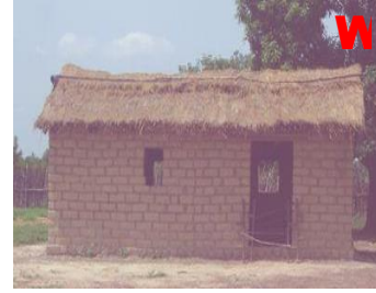
concrete houses geo mounted with cement
