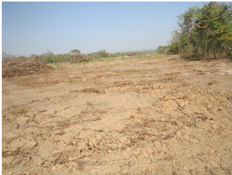
Photo 1: View of the runway site
